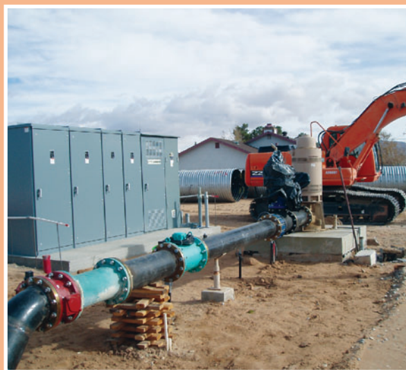
Pictured at right: Well 11R Site Improvements
