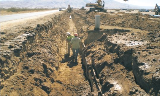
Installation of approximately 1.5 mile of 12" water main Central and Sandia Roads improves water distribution capabilities and fire flows.
