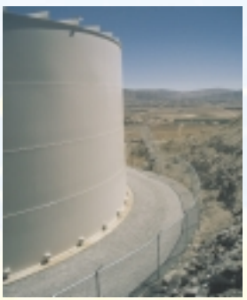
New Corwin Tank Reservoir
