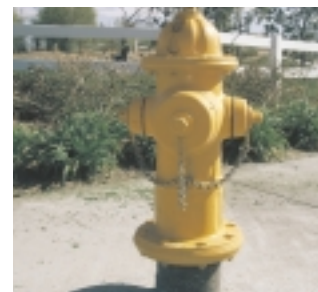
New four-way fire hydrant
