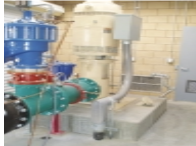
A newly commissioned water well.
