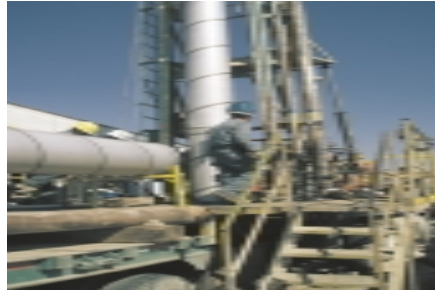
Well drillers install the well casing at new well #36.
